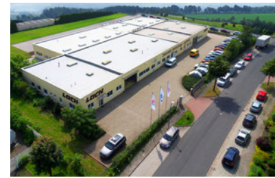
Plant in Lichtenau near Chemnitz, Germany
